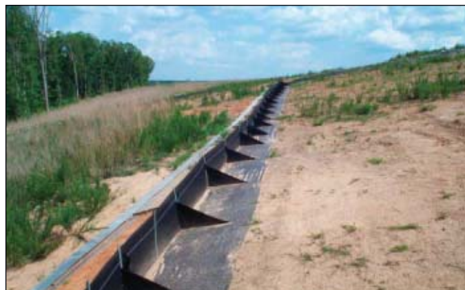
Researchers installed Failure Avoidance Effective Silt Fence Technology on a landfill site in Greenville, SC (Fig. 2).
