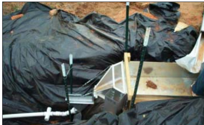
An H-flume calibrated to measure flow rate measured discharge through the fence before diverting a representative portion of the discharge and sediment to a collection tank (Fig. 4).
